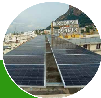
Soorya Multispecialty Hospital 40 KW, Tiruchengode
